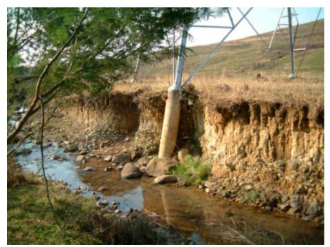
Figure 8. Example of the dangers of erosion to power lines (photo Jorge Correia)
